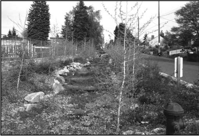
Bioretention facilities alongside streets capture runoff and prevent pollution from entering the Sound through stormwater systems. | Photo by Bruce Wulkan
